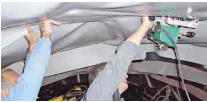
Comet operating in the tunnel ...
