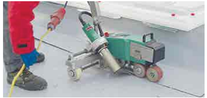
Due to its slimline design, welding is possible even up close to edges.
